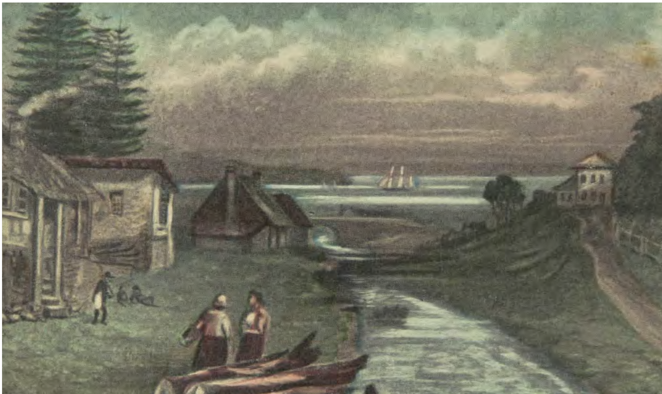
62. Tank Stream, Old Sydney - when a severe drought reduced the stream to a little trickle, three tanks were excavated from the sandstone, giving the stream its present name.
